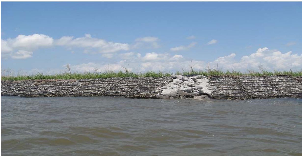
Revetment lined shoreline. The rock pile indicates a "turn" in the shoreline.
